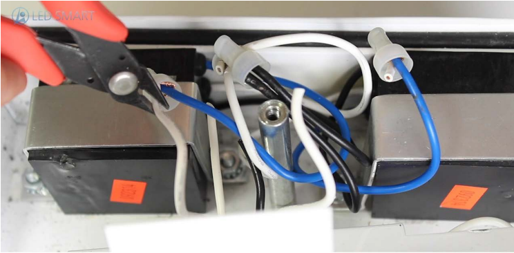
10. Cut all 4 wires that are coming out of the bottom of the lamp holder support bracket
