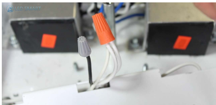
13. Put wire nuts on exposed wires
