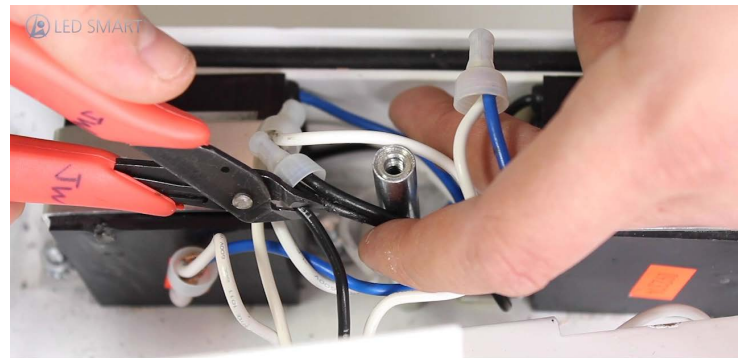
10. Cut all 4 wires that are coming out of the bottom of the lamp holder support bracket
