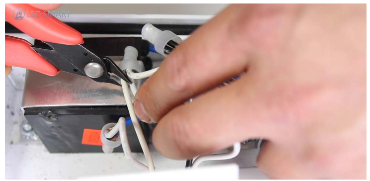
10. Cut all 4 wires that are coming out of the bottom of the lamp holder support bracket
