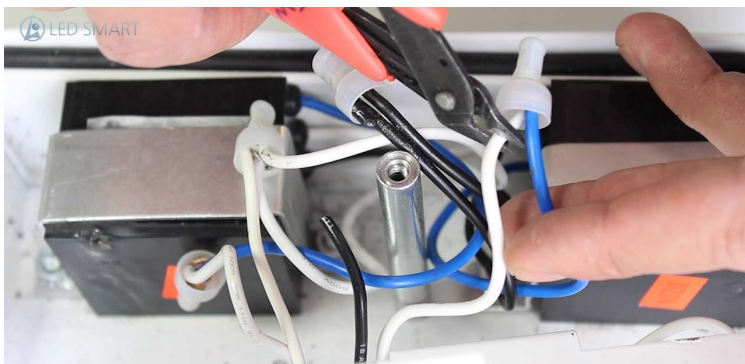
10. Cut all 4 wires that are coming out of the bottom of the lamp holder support bracket
