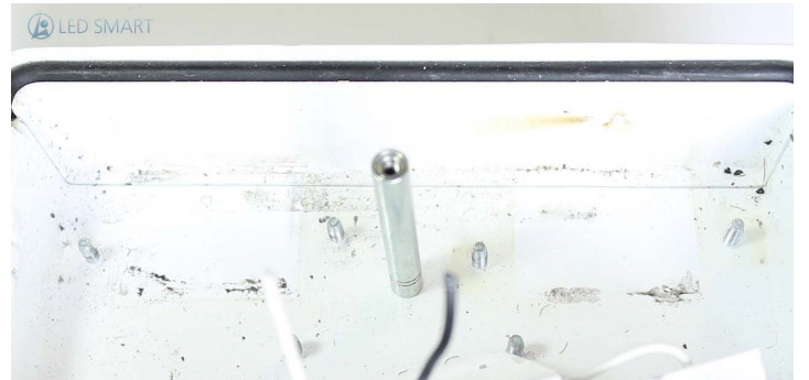
11. Remove the nuts from the ballast cases and remove the ballasts
